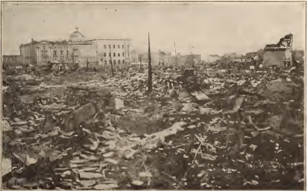
YOKOHAMA SPECIE BANK BUILDING, STANDING BUT IN RUINS (G. W. R.)
